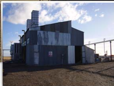
La Marina Compression Plant
